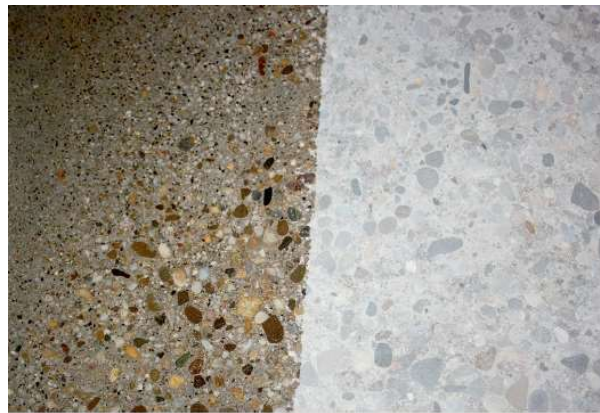
Figure 2. The diluted thin-layer coating agent was applied to the sanded-down concrete floor [4]
